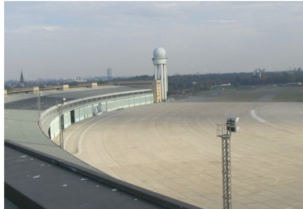
The view of hangars from roof, facing east. Photo: Alex Lawler, Courtesy the Artist.
